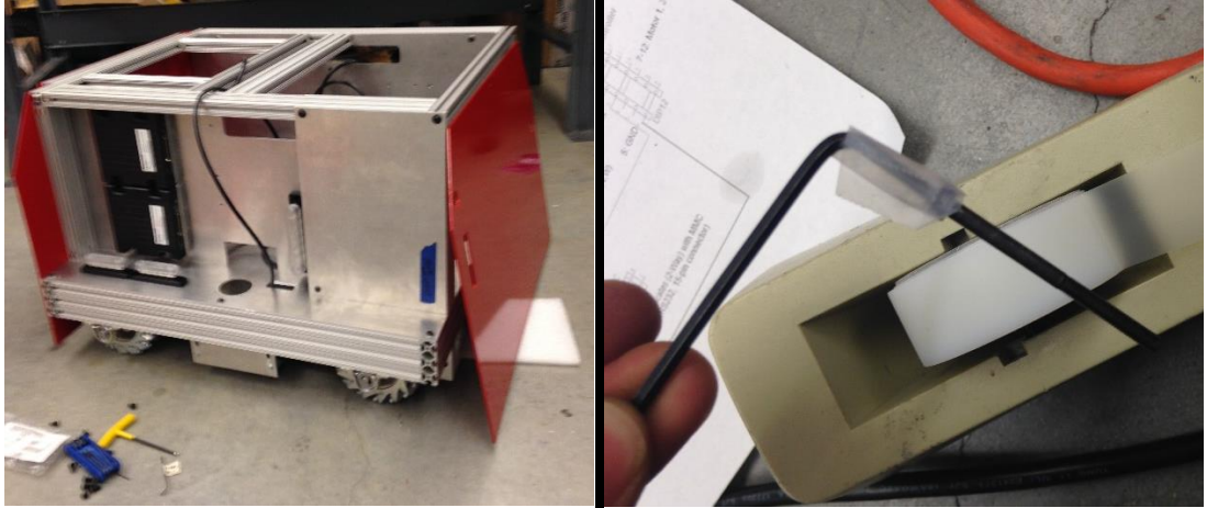
Figure 26. Left: Some plating, bus bars, and electrical components added. Right: get creative. Sometimes taping a screw onto an Allen wrench aids in adding a difficult screw.
